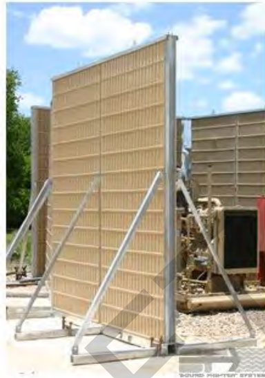
Figure 9.3: Example of a Section of Temporary Noise Barrier
