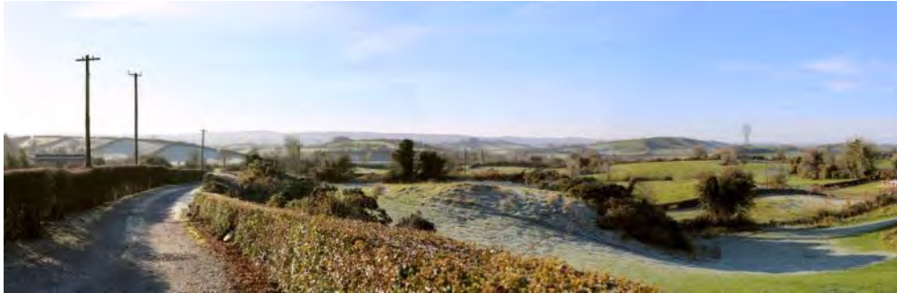
Photomontage 12 from local road L7411 at Drumroosk townland at a distance of approximately 535m. This represents an open view from an elevated location over a landscape of dense drumlins. Six towers are partly visible, travelling into the distance, a further four are screened by topography.
